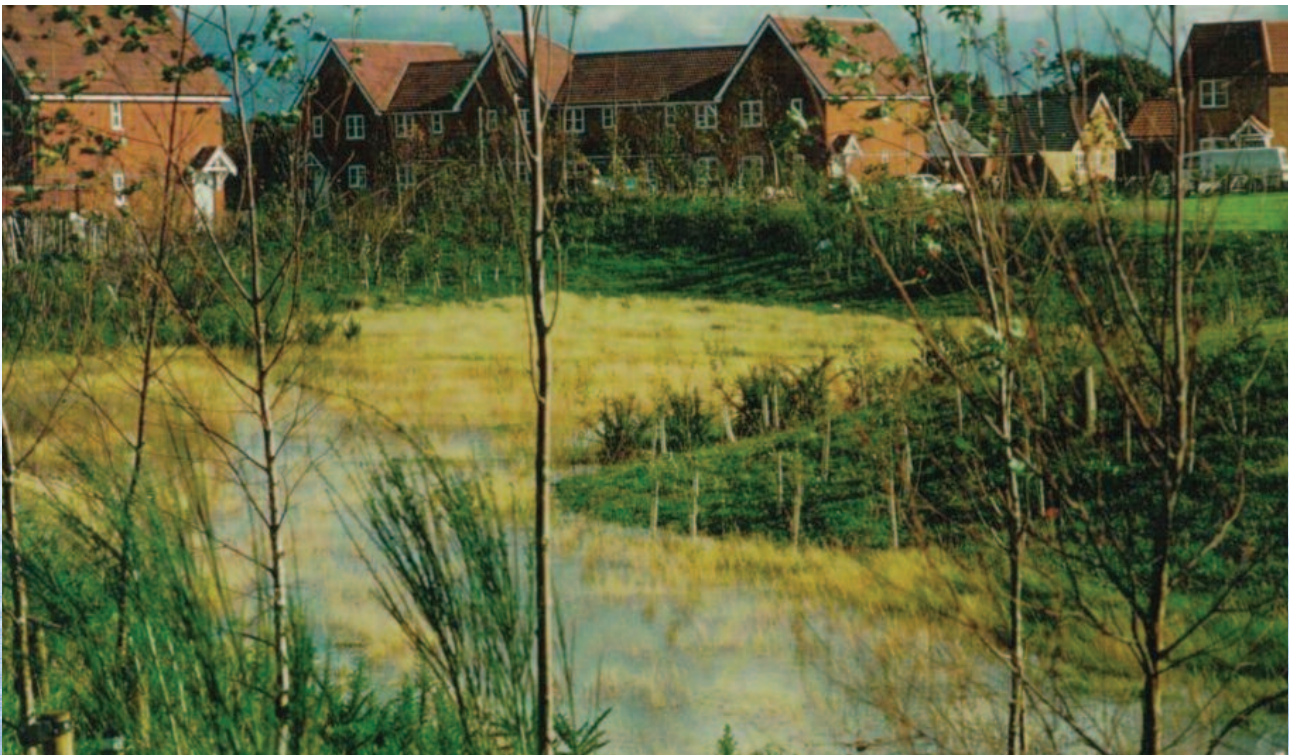
Sustainable drainage system in Ipswich
