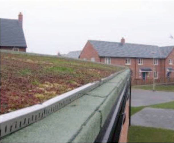
Green roof on a shed
