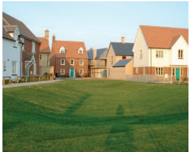
Infiltration basin in dry state, Ipswich
