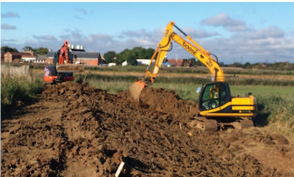
Repairs to flood bank
