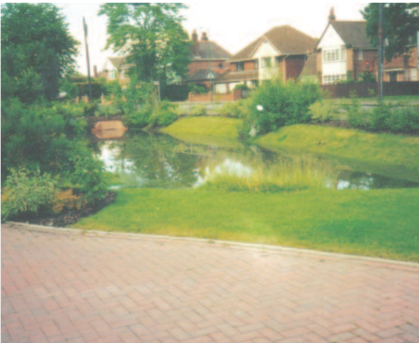
Detention Basin, Ipswich
